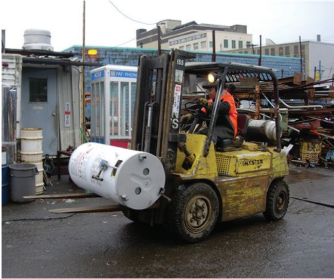
Mandatory recycling at demolition and construction sites.
